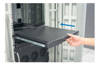
Press the handle button and gently push back the drawer into the rack.
