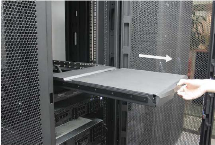
Figure 4. Sliding out the LCD keyboard drawer by pressing the carry handle button first.
