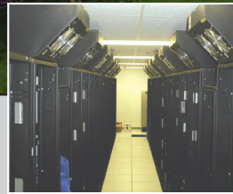
Inset: Liebert XDV units installed on the racks of the Virginia Tech supercomputer.
